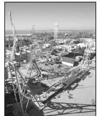
Figure 3: Wicked Twister under construction.
